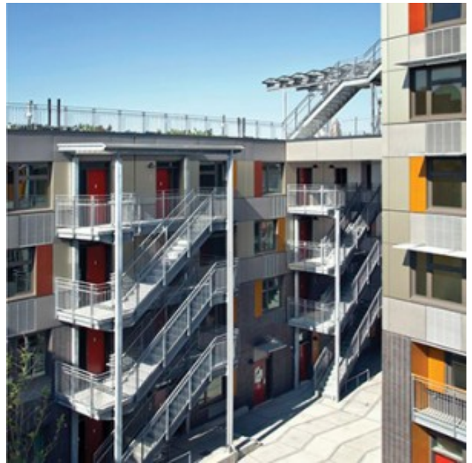
Codeveloped by Jonathan Rose Companies and Phipps Houses, Via Verde is on a 1.5-acre (0.6 ha) site in the South Bronx in New York with access to mass transit. The mixed-use project serves a range of income levels with 151 rental apartments and 71 co-ops. Connected green rooftops provide access to garden plots and open space while stairs are incorporated throughout the project. (David Sundberg)
